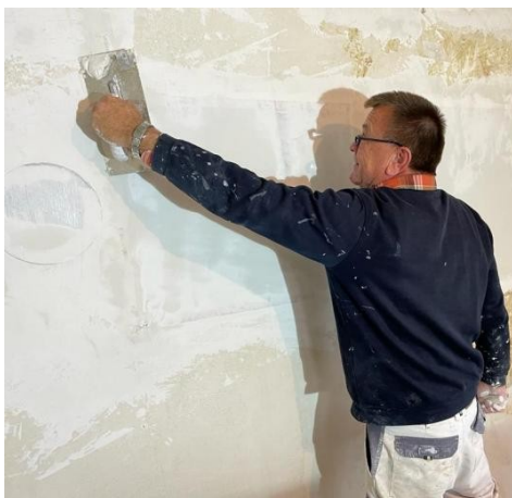
P23 Applying Plaster Top Coat
