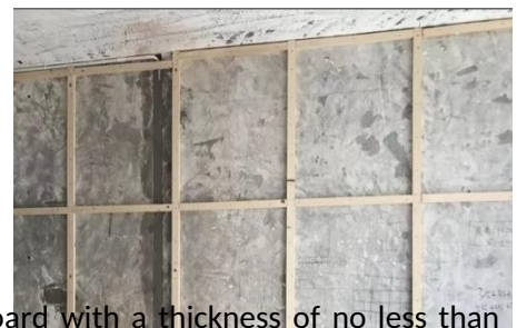
P13 Wooden profiles for installation of insulation
