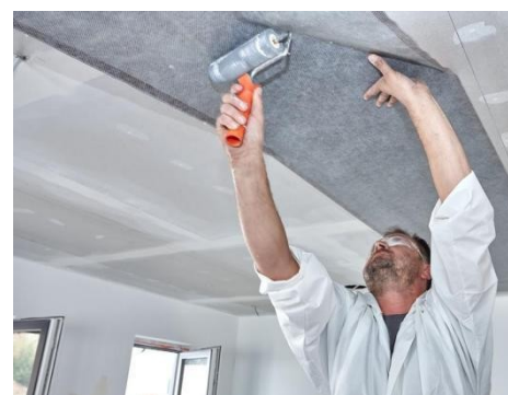
P21 Pressing the heating film using a roller
