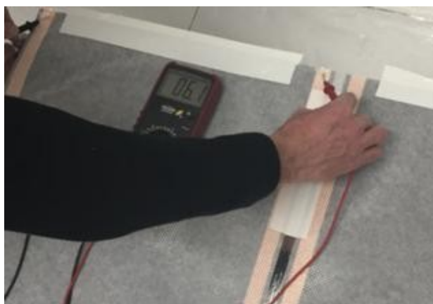
P 9 Test the heating film resistance
