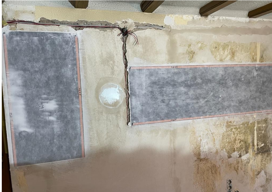
P 22 Treating the wiring slot
