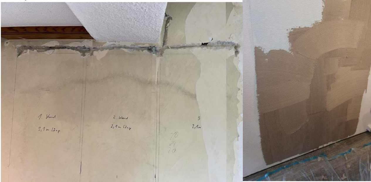
P3 Preparing the installation surface
