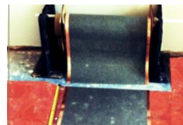
P17 Cutting the heating film (Manual cutting can be done for smaller projects)
