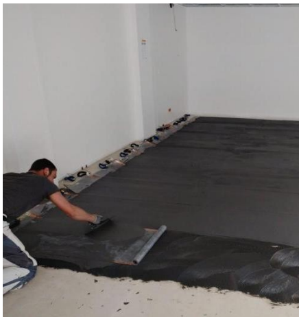
P6 Cement mortar surface installation
