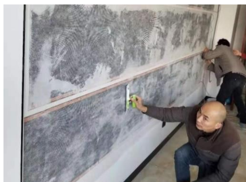
P20 Pressing the heating film into the plaster
