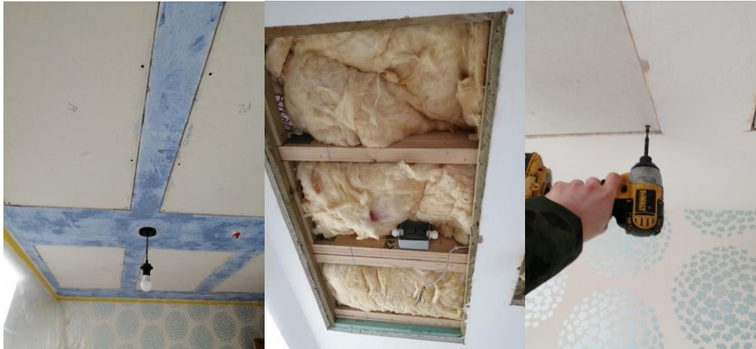
FIG 3:POWERBOARD S INSTALLATION
